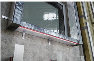
Where access constraints mean brackets cannot be fixed above the cavity barrier, brackets can be fixed beneath the horizontal barrier.
