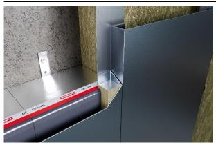
1. If the panel depth is bigger than the barrier allowed air gap, notch the barrier around the cassette panel return.
