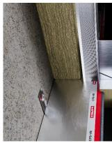
Always ensure the distance between the back of the panel and the edge of the barrier does not exceed the maximum air gap the barrier can accommodate.
