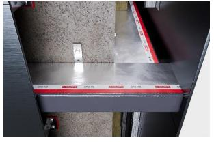
Ensure there is no gap between the cladding and the edge of the oversailing barrier.
