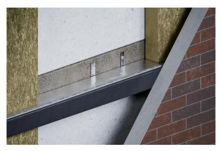
Build brickwork up to the slab level and then install the non-ventilated barrier to the slab.
