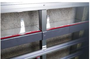
Alternatively, when the façade rail partially intersects the leading edge of the barrier, notch the barrier to accommodate the rail and fix the intumescent material to the front of the rail.
