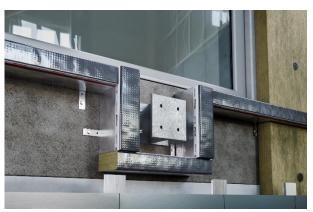
When the cavity barrier line is interrupted by balcony brackets, encapsulate the balcony brackets with non-ventilated barriers vertically, and ventilated barriers horizontally.
