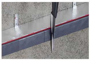
Make an incision into the intumescent material of CFS-VB, at the edge of the panel return, to ensure the barrier can freely expand into the cassette.
